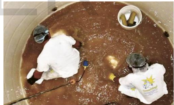
Fig1.1 Manual cleaning of water tank
